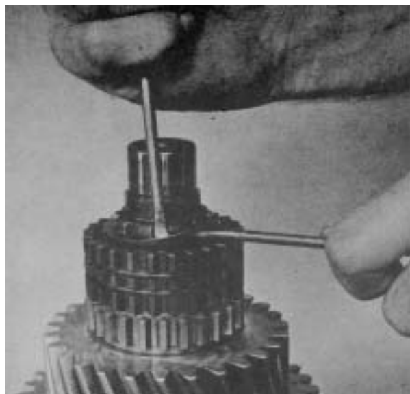
Figure 25 - Remove 4th & 5th shift hub sleeve retainer ring.
