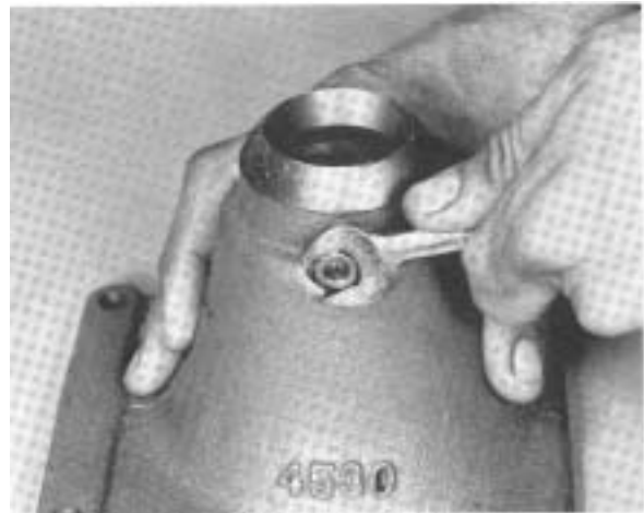
#148 - Installing nut on gear shift lever pivot pin.
