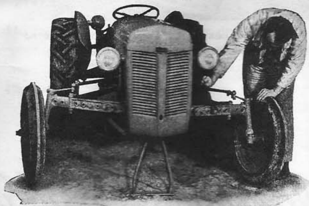
Adjusting front wheel tread width.
