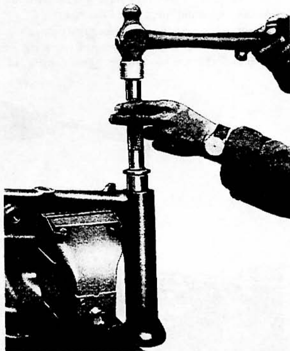
FIGURE 6 FITTING NEW SPINDLE BUSHES
