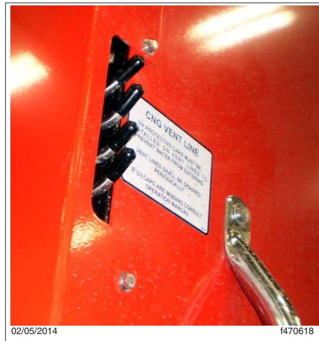
Fig. 21.9, CNG Vent Line Caps
