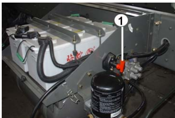
1- Master power switch
