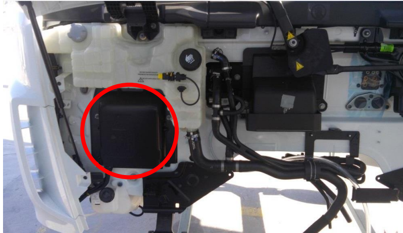
Figure 7-3.1 Electrical Junction Box Location
