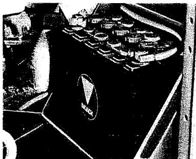
Battery negative cable
